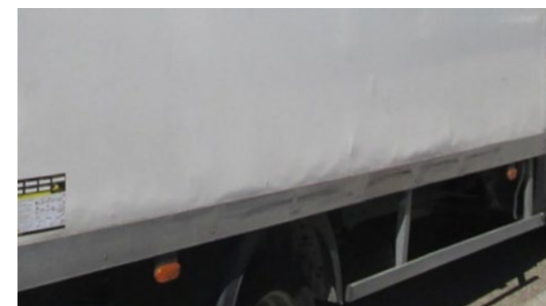
Fibreglas side panels: Deformation on lower part, length of > 1\text{ m} NB: Replacement of the front panel of the underbody requires removal of the underbody.
